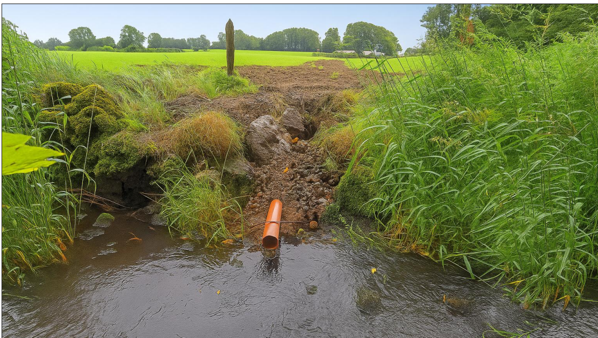
Plate 4.6 Recently installed land drain at site B2 on an unnamed River Robe tributary, July 2025
